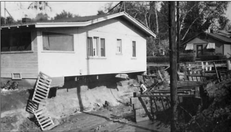
F. E. Montee of 4815 Avoca Street, whose house was undermined and the front yard washed away to the front doorstep, said "Tell them for me that we need the Yosemite storm drain system. I hope we get it." (photo ERVHS Archive)
