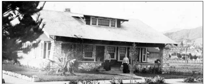
The house at Maywood and Fair Park which Ferdon built for his parents Clay and Mellissa. Gates Hall was then directly across Maywood Avenue.
